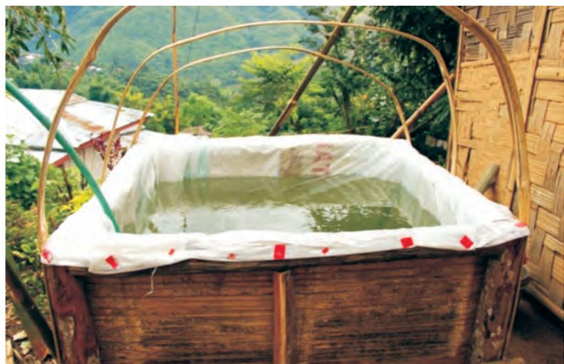
and Northeast in general, where there is plenty of bamboo. The average life span of each bamboo made structure is expected to be 2-3 years.
